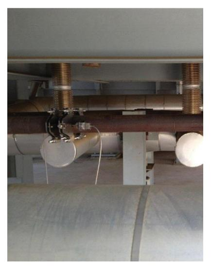
Smaller does not mean easier. Engineers got creative and used noise levels to determine whether water or steam was passing through the 2-inch drain pipe. Courtesy: FLEXIM Americas
